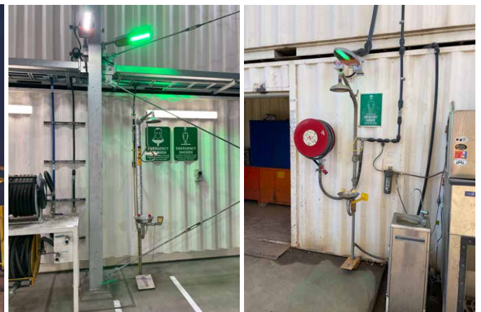
ABOVE & BELOW: Mako Area lights and Mako Emergency lights, mounted on Swivelpoles around the walkways, stairways and gantries. 480W MegaFloods with trunion brackets, mounted on poles above the walls, accompanied by Silverback 40W IK10 IP66 batters mounted on walls and under walkways. BELOW RIGHT: Emergency Eyewash Stations featuring Green LED Mako Area Lights.
